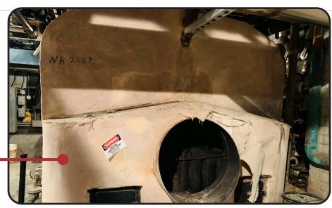
PHOTO 4: PREVIOUS BOILER W/ ASBESTOS WARNING
