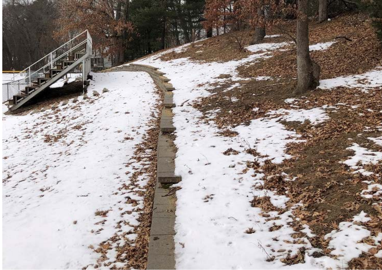
View from Retaining Wall – Bleachers
