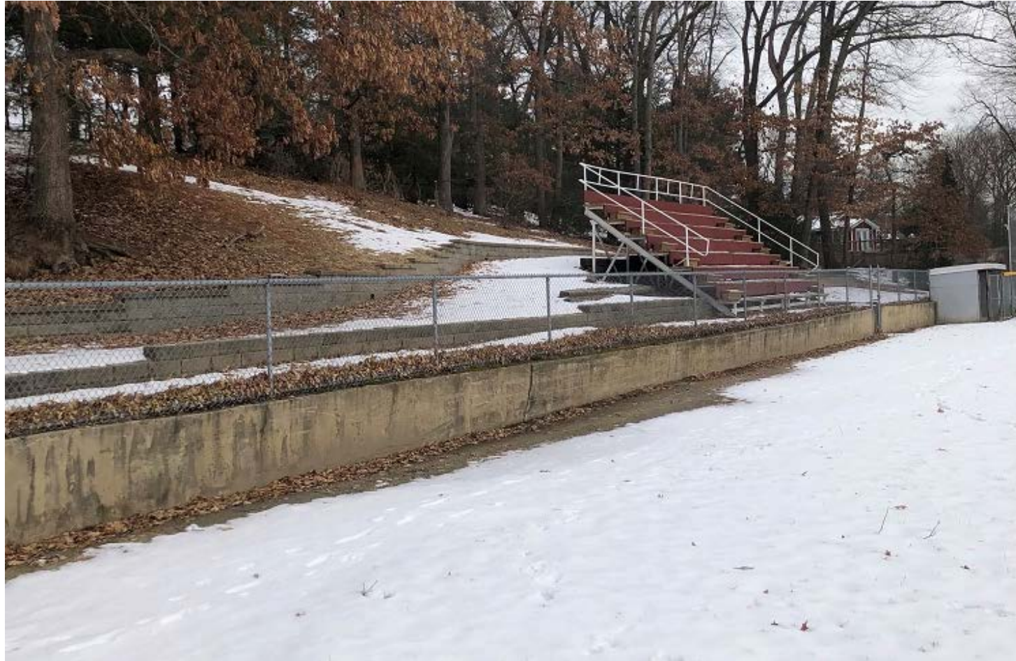
View from Lions Field – Retaining Wall & Bleachers
